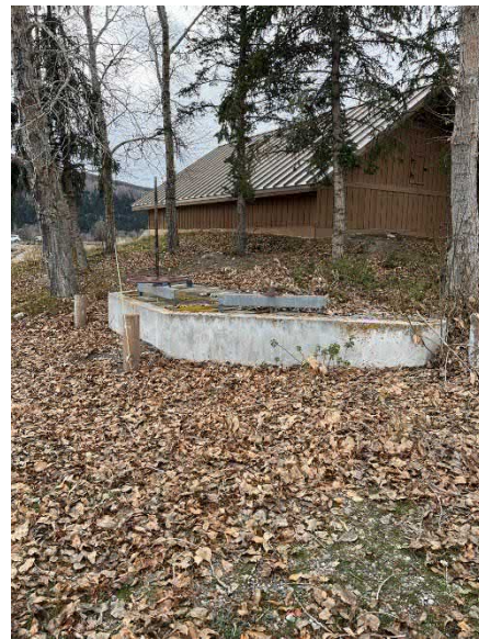
Photo 1.27. Cell 4 Water Control Structure
