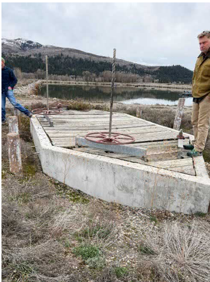
Photo 1.26. Cell 3A Water Control Structure
