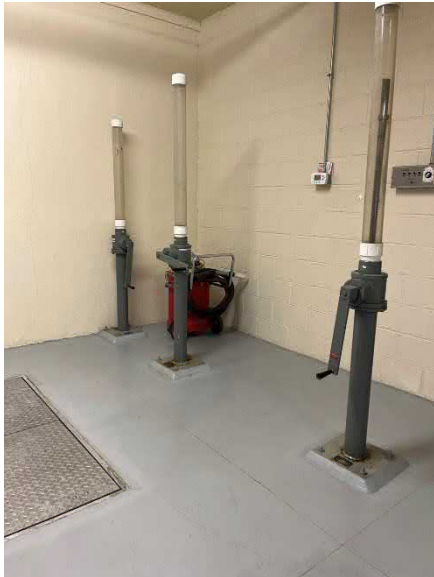
Photo 1.28. Cell 5 Water Control Structure
